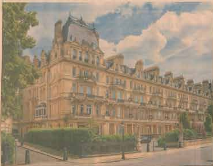
Apartment block on Cassette Terrace where a three-bedroom, flat has apartment it was sold for £200k
